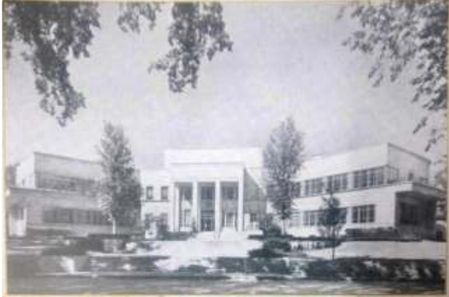
Rotary International Headquarters (old office) at 1600, Ridge Avenue, Evanston, Illinois.
